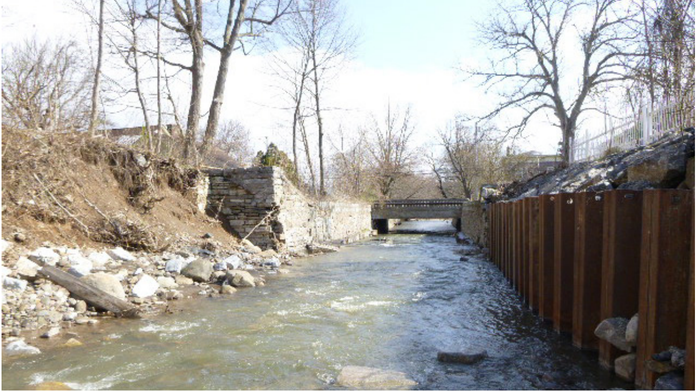
Photo 24: Retaining walls along Moyer Creek in the Village
