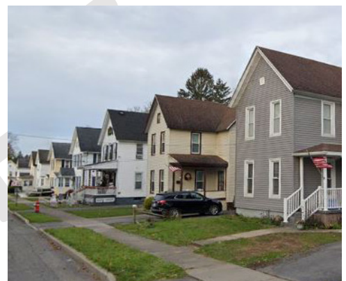
Photo 4: Houses on Fifth Avenue Source: Google Street View
